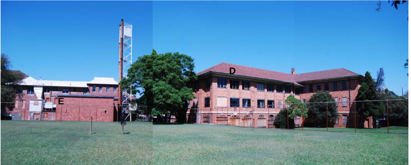
Figure 5: View from the north with the old Boiler Room (E) on the left and the Dormitory (D) on the right. (GAO 2008)
