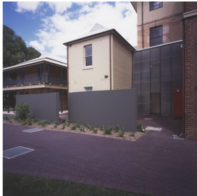
Figure 12: Existing paved pedestrian / vehicle route in front of Building B in alignment with proposed right-of-way.
