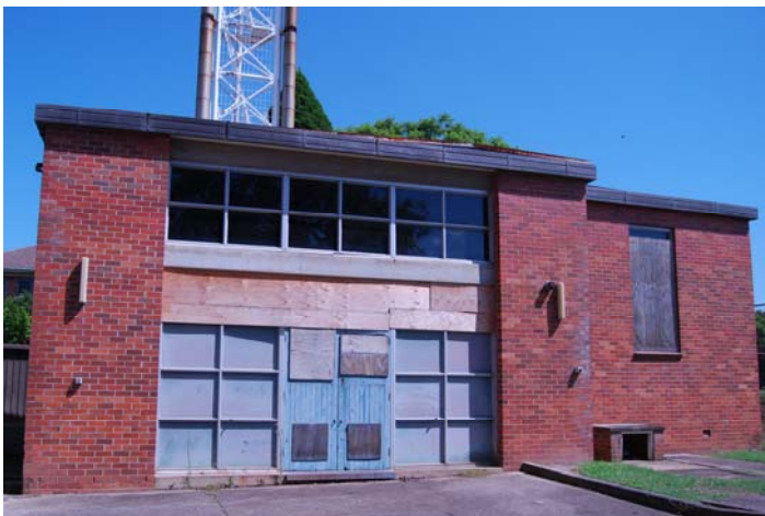
Figure 8: Eastern elevation of the Boiler House (Building E).
